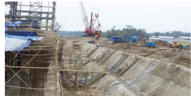
PROTEKSI MEMBRAN KOLAM WATER TREATMENT - TANGERANG
